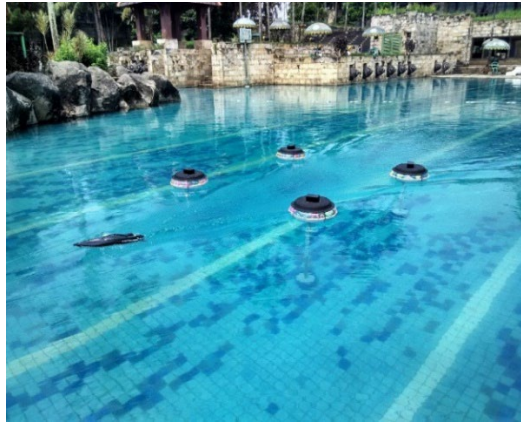
Figure 8. Sensor setup in pool water.
