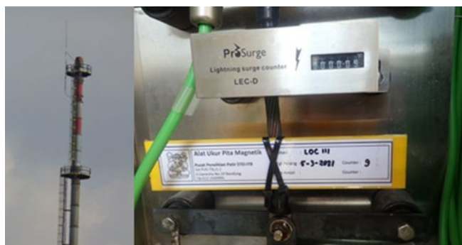
Figure 6. Installation of measurement system in Cilacap stack structure
