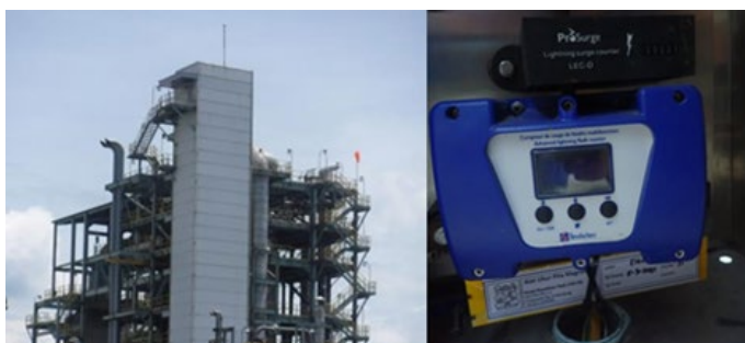
Figure 7. Installation of measurement system in Cilacap refinery structure
