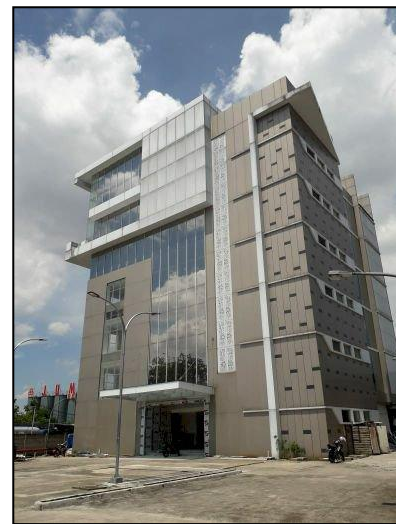
Yos Sudarso Building, North Jakarta. Latitude: 6°7'18.89"S, Longitude: 106°53'34.42"E.
